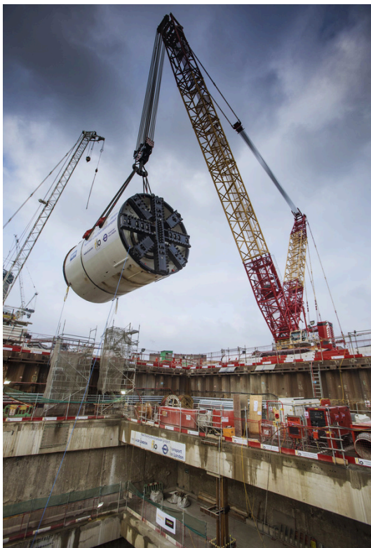
Northern Line Extension – TBMs Instalados.
