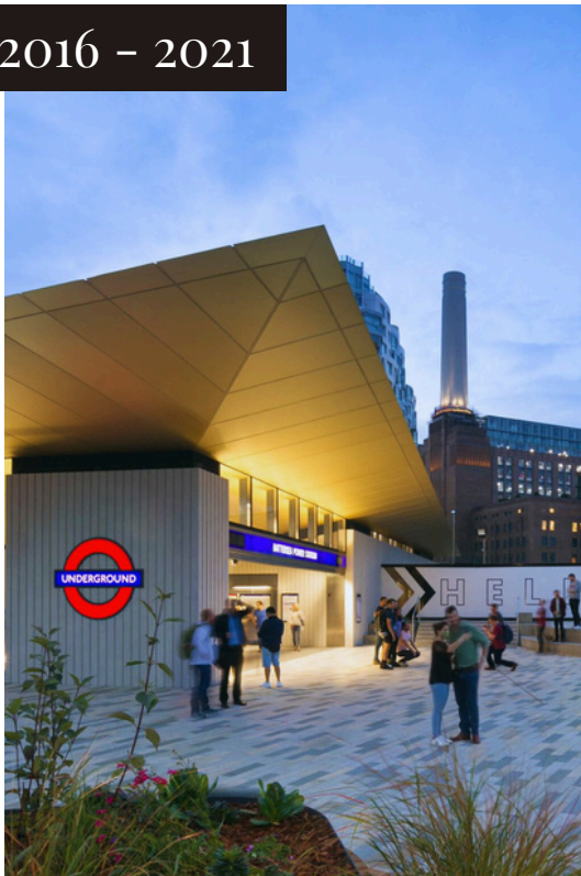
Northern Line Station - Battersea.
